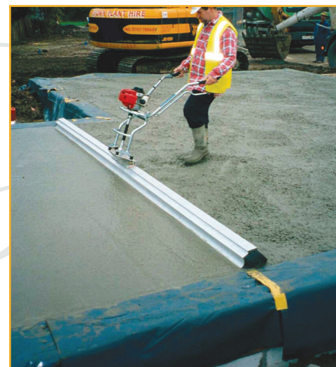
Free Screeding and form work screeding possible
